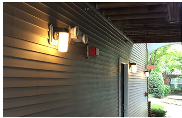
Interior Hallway-Installed LED Lights
